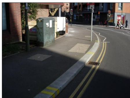
PHOTOGRAPH 4 EXISTING VIRGIN MEDIA CHAMBERS AND CABINET IN FOOTWAY ADJACENT TO BUILDING FRONT ENTRANCE
