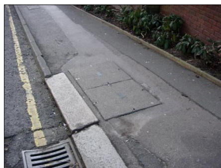
PHOTOGRAPH 2 EXISTING BT CHAMBER ADJACENT TO BUILDING IN FOOTWAY ON WARWICK ROAD
